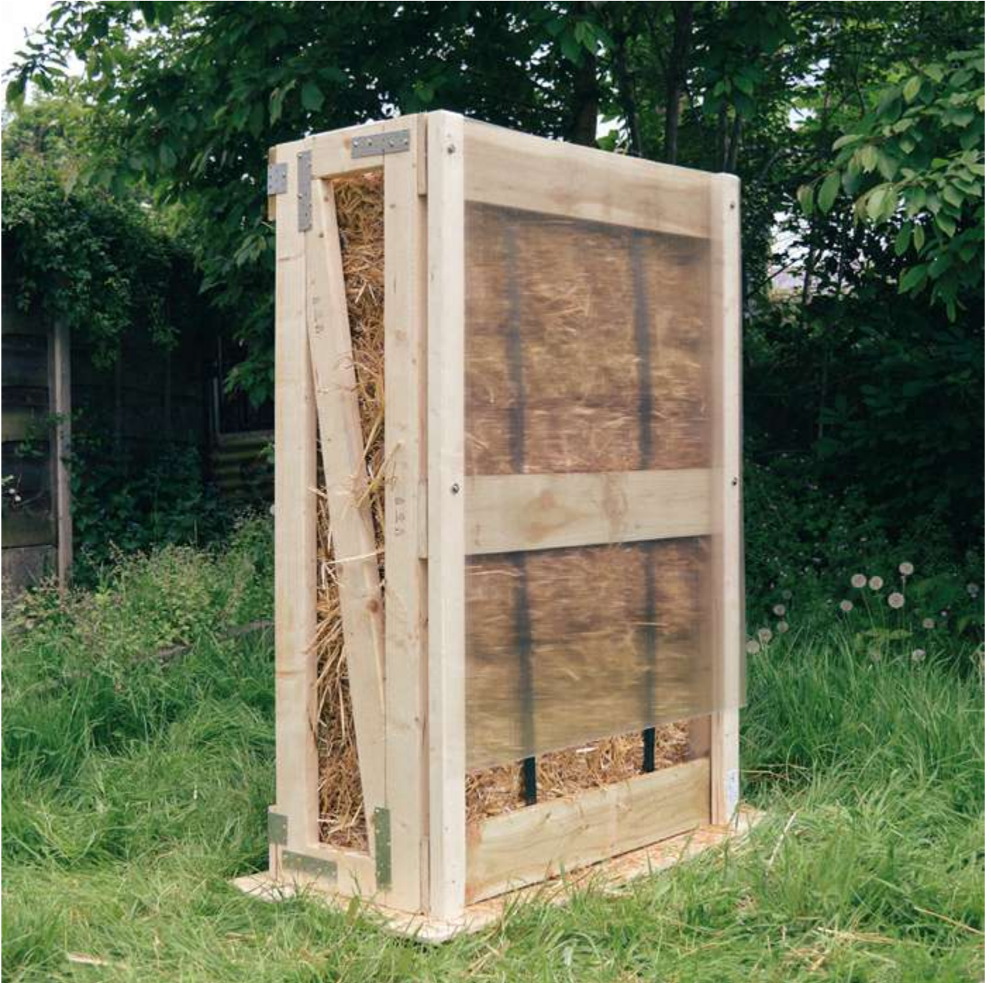
1:1 co-built straw and low grade timber module prototype constructed with the support of unskilled volunteers.
