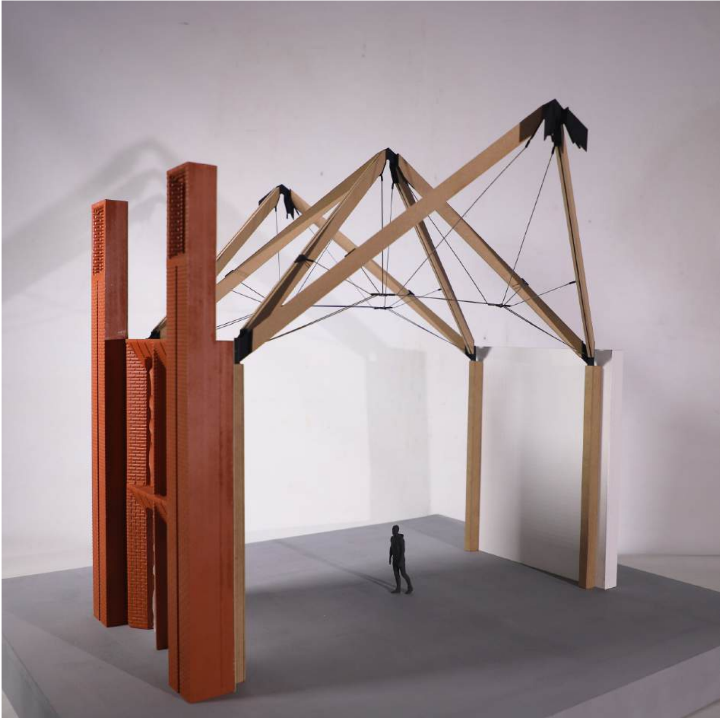
Cover Image: Photo of a 1:20 structure model showing a multifunctional hall's network-like structural system with bespoke 3D-printed junctions, MDF laser-cut beams, and 3D-printed tension bars with metal wires. This design, refined with a structural engineer, enhances stability against various loads while promoting sustainability and efficient space use.
