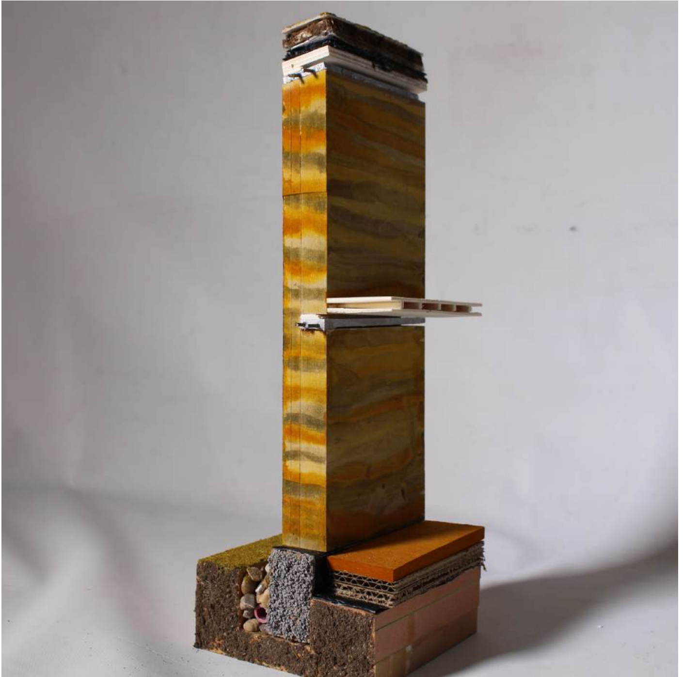
Detail on the gravel drainage and stone foundation.
