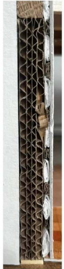
Image 15: External wall section
