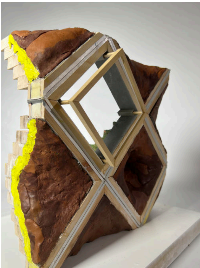
Image 06: The image on the left provides an interior view of both the model and the actual building. As depicted in the model, the operational windows feature a parallel projectile design. Additionally, the cut section reveals the various components used for insulation, including foam as the insulation material, black-colored paper acting as a breather membrane, and timber panels serving as the structural frames. Notably, the interior of the parametric cladding is showcased as a smooth surface, in contrast to the exterior cladding. This distinction is a result of the driving motivation behind my work in Studio 3.1 and 3.2, along with the subsequent development and enhancements made from the initial Studio 3.1 project to the refined Studio 3.2 project.
