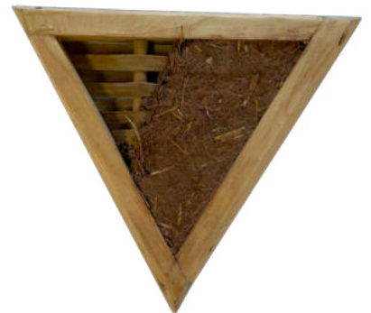
Images 5&6 (L&R Respectively): 5) Wattle and Daub build up, staves, reeds, earth and plaster finish, within a darkened timber frame a la tudor frame constructs. 1:1 Section 6) Triangular Wattle and Daub Module for various geodesic forms 1:10
