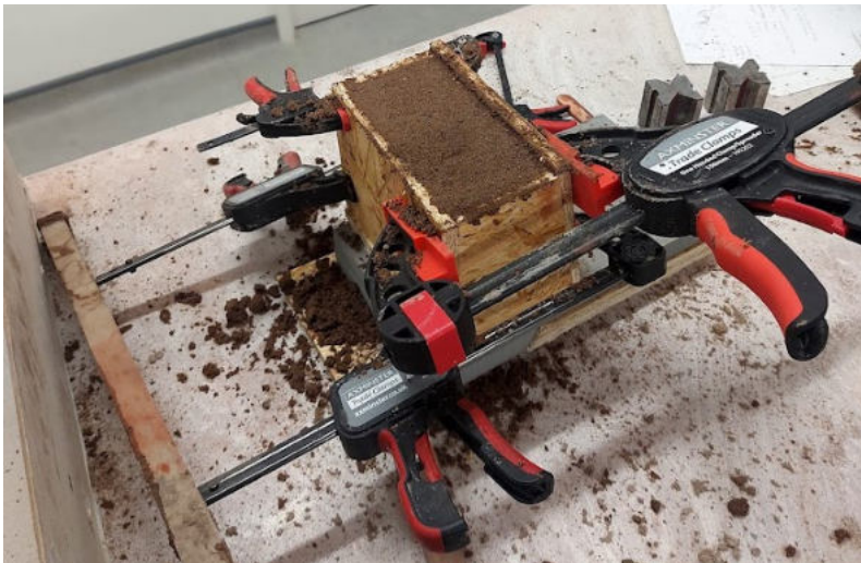
Image 05: Rammed earth wall construction Chipboard former held in place with clamps as I rammed the earth
