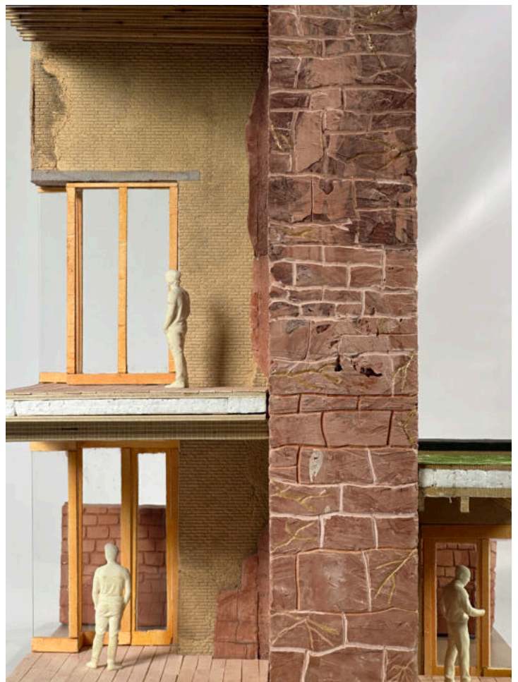
Image 02: The technique of Kintsugi to represent how they stabilised and repaired the existing wall
