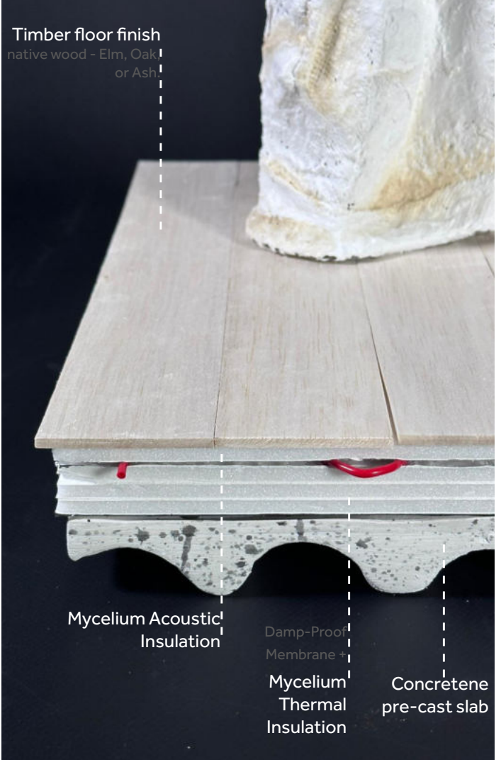
Image 04: Detail of materials in the floor buildup
