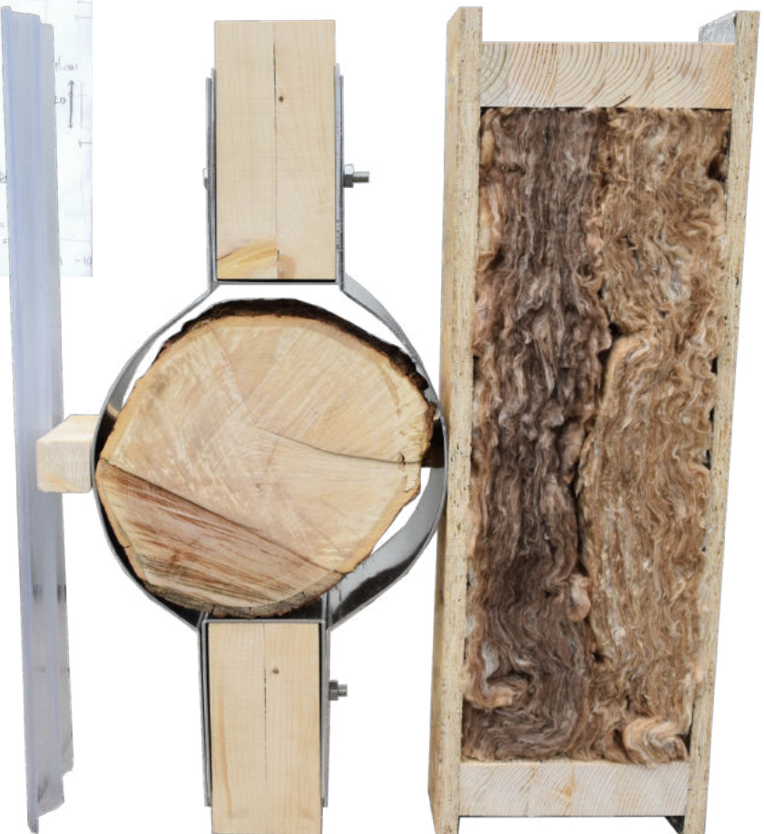
Image 05: 1:1 detail model (developed alongside 1:10 model): scavenged corrugated polycarbonate, scavenged timber studs, 3mm aluminium, steel bolts/nuts, scavenged cherry tree log, OSB, scavenged ecobatt insulation
