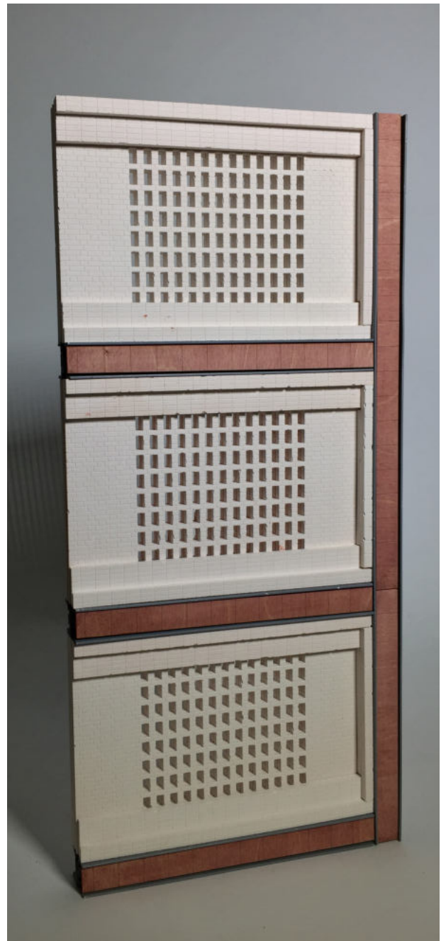
Image 05: 1:20 External Facade Model- Plaster cast elements, steel frame with stained plywood inserts.
