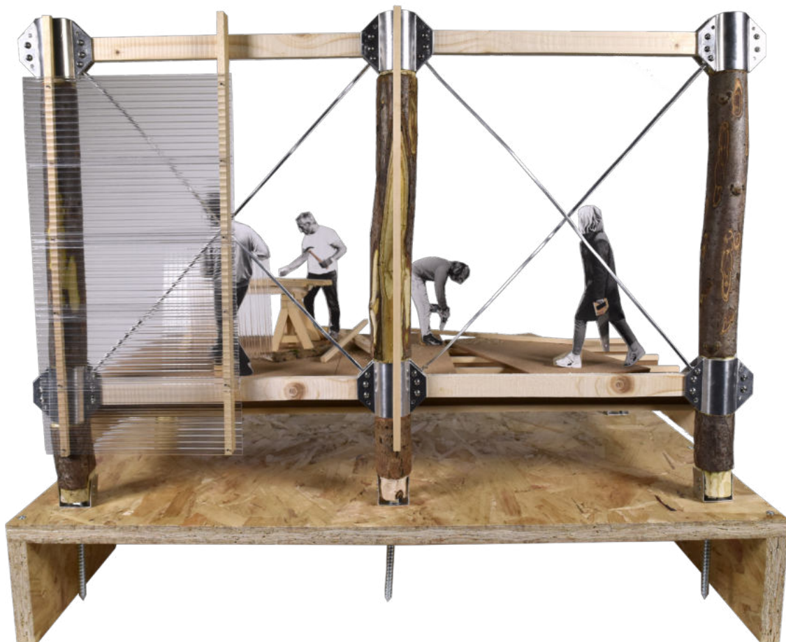
Image 01: 1:10 facade detail model: cherry branch, aluminium, steel bolts/nuts, OSB, cork, timber studs, corrugated styrene
