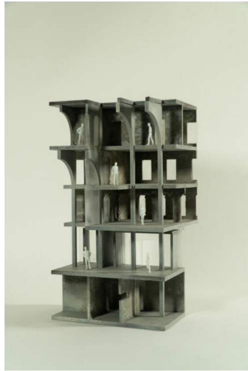
Image 04: Prototype 2 Corner Model 1:200 Scale 2mm MDF Perspex sheet Acrylic block Mahogany Stained Mahogany
