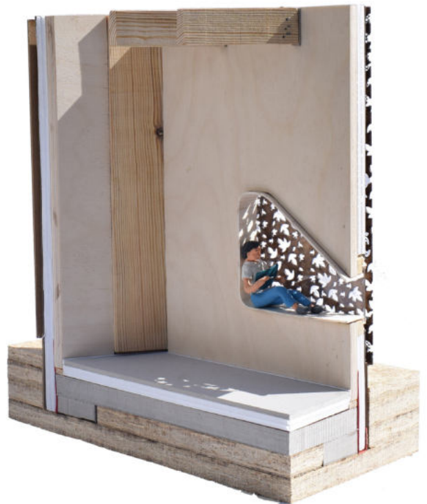
Image 06: Detail model- Wood, foamboard, greyboard, metal mesh, card, plasticine person
