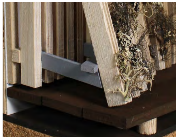
Image 3: Steel structure connecting the two layers of cladding - detail
