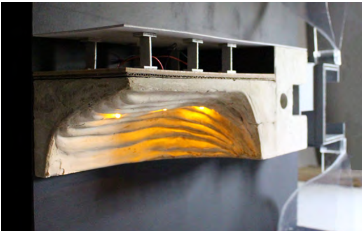
Image 02: Showing layers, hollowed out form with the access floor on top and ETFE facade to the right.
