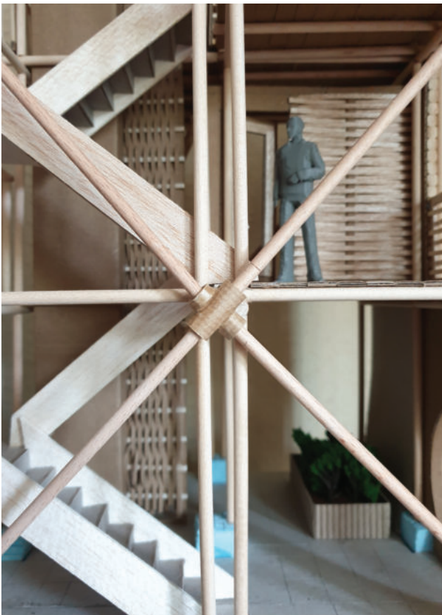
Image 02: Physical Model (Scale 1:20) - Cross-bracing node detail
